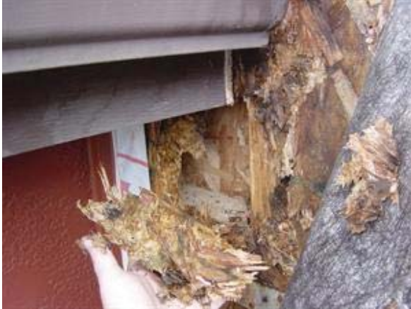
Roof and siding protection
